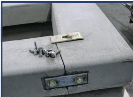
SPLIT PADS FOR REPLACEMENT
