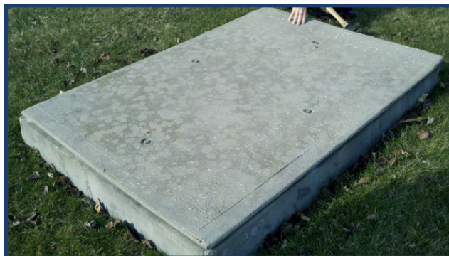
For safety and security reasons, covers are used in delayed equipment installation; where the box pad is installed prior to the electrical equipment.
