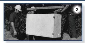
If the ground sleeve is not assembled in the excavated hole, it's placement can be done in one of two ways. Small lightweight units can be placed by hand. Larger units my need hoisting equipment.
