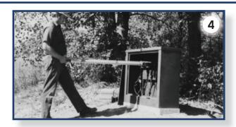
Center the electrical equipment onto the ground sleeve. Using the provided hold-down C-Clamps, attach the equipment to the top flange of the ground sleeve.
