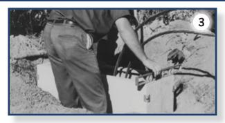
Once the ground sleeve is in the desired location, check to ensure that the unit is level, and that the entire bottom flange is supported equally. Then backfill the hole to the desired grade level.
