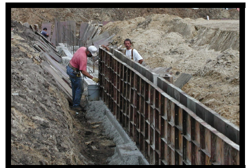
Assembling the footing forms.
